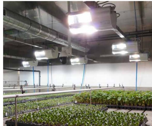
**At Semillas Fitó, two germination chambers have been updated with a total of 18 new 250 W LED lamps, replacing the incandescent halide lamps which consumed 315 W each.**
